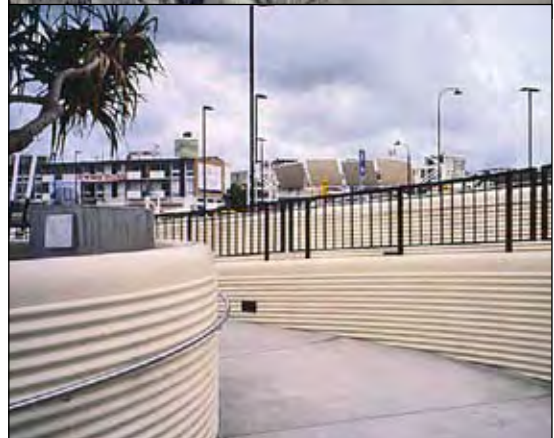
Figure 8: Examples of formliners used to create decorative off-form finishes
