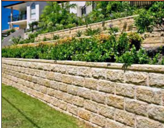
Figure 5: Examples of reinforced concrete masonry cantilever retaining walls
