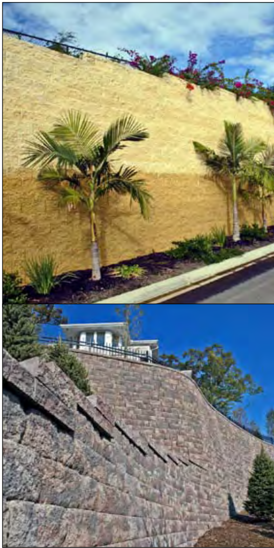
Figure 12: Examples of segmental concrete reinforced soil retaining walls
